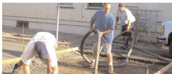
New driveway is poured
