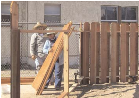
Elena & Tony work on fence
