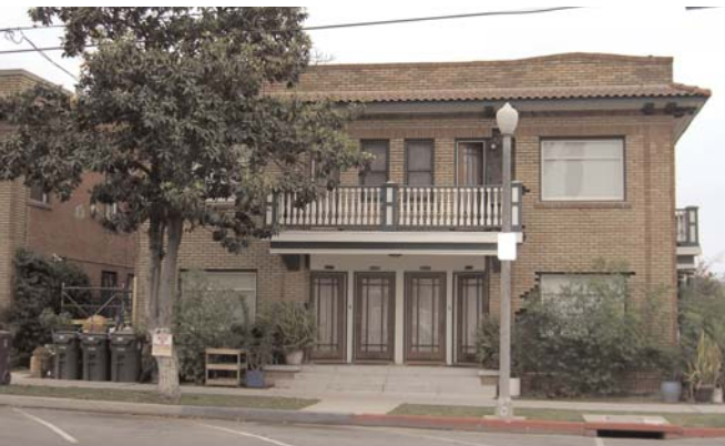
All of the bricks are being removed and reinstalled
