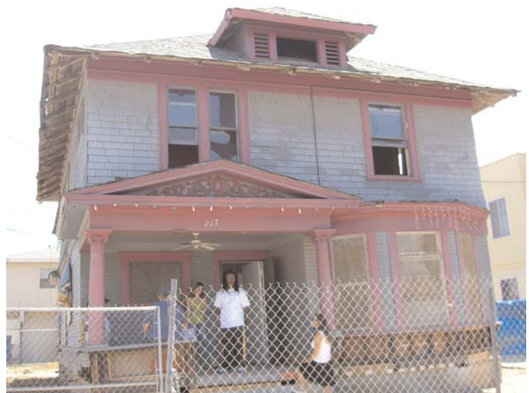
226 W. 10th Street American Foursquare style built in 1905
